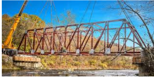
Figure 5.11: An example of through-truss steel bridges.
